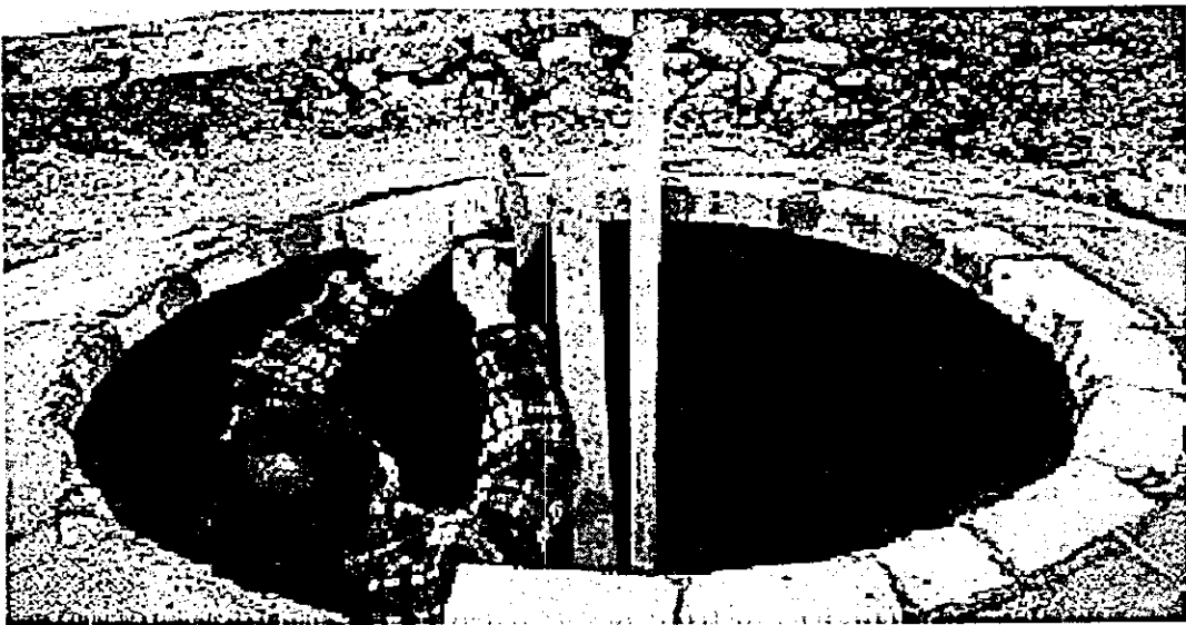
Fig.3: Fixed-dome plant in Tunisia. The final layers of the masonry structure are being fixed
