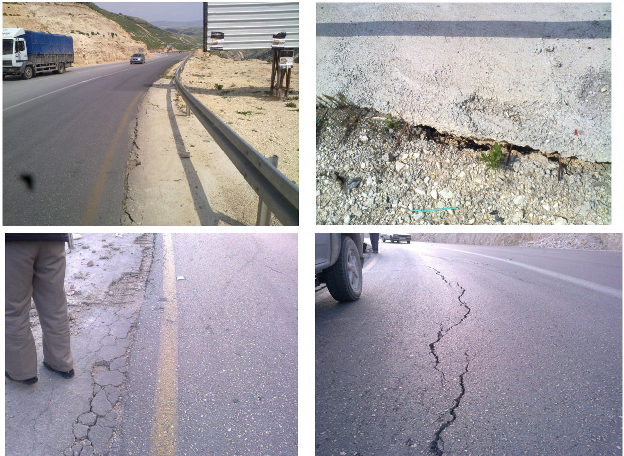
Figure 1: Typical cracks that occurs yearly along Nablus – Al-Bathan Road.
