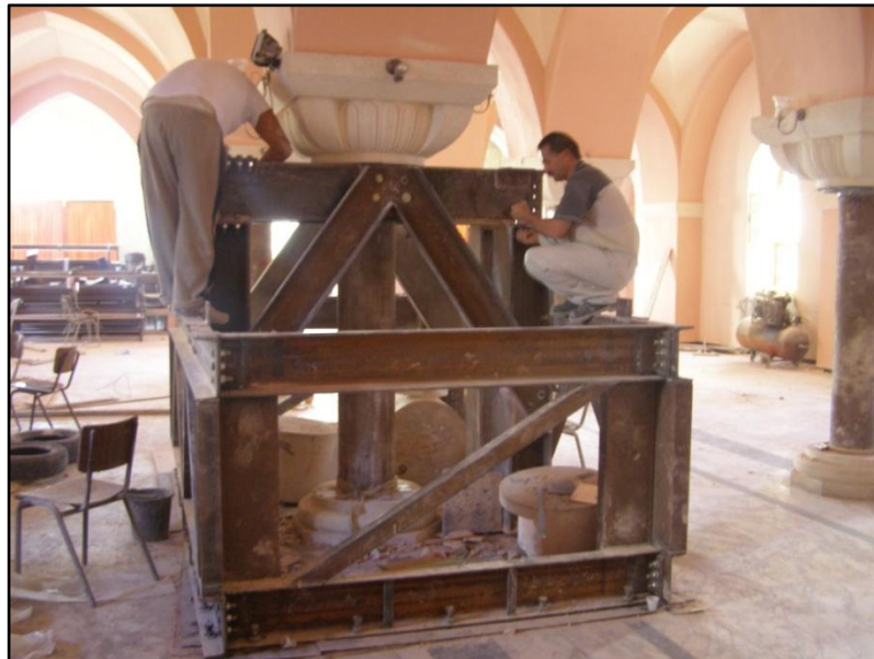
Photo 4 The Shoring Steel Frame
