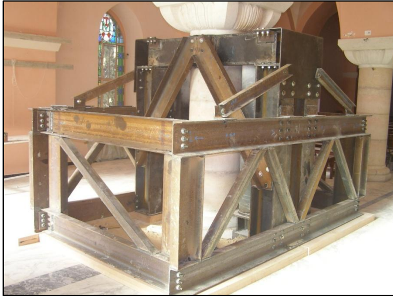
Photo 3 The shoring steel frame
